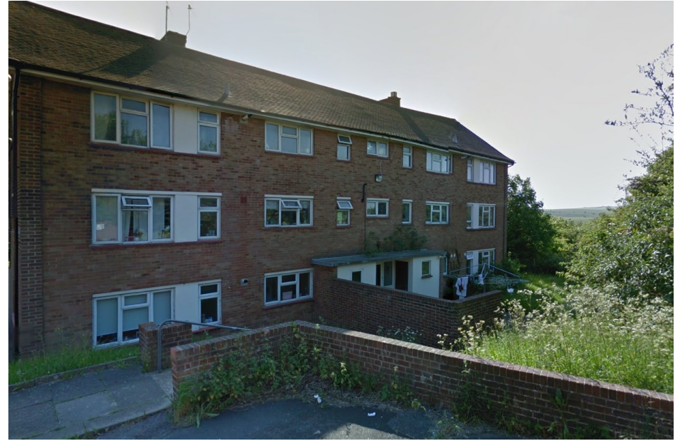
4. Flats opposite the garages in Buckley Close
