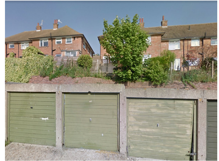
2. Existing garages and rear of properties in Chichester Close
